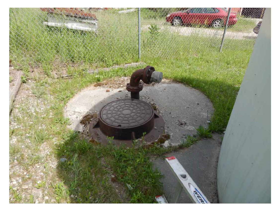
EXISTING BY-PASS MANHOLE PHOTOS SCALE: NOT TO SCALE
